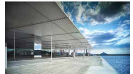
KAZUYO SEJIMA + RYUE NISHIZAWA / SANAA "Marine Station "Naoshima"
